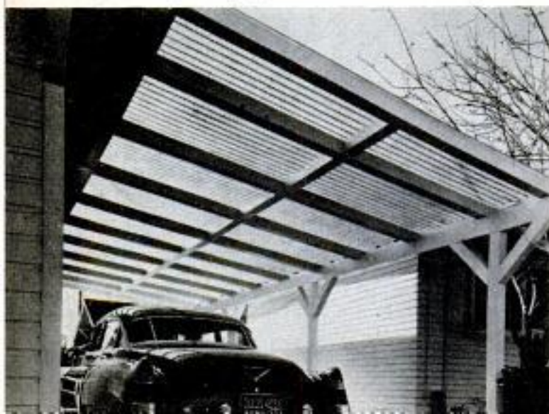
Alpyrite Company of America photos Above, flat-type translucent plastic may be used in place of regular frosted glass where vision is not desired. Below, panels of corrugated plastic, 10 or 12 ft. long, simplify construction of a carport roof
